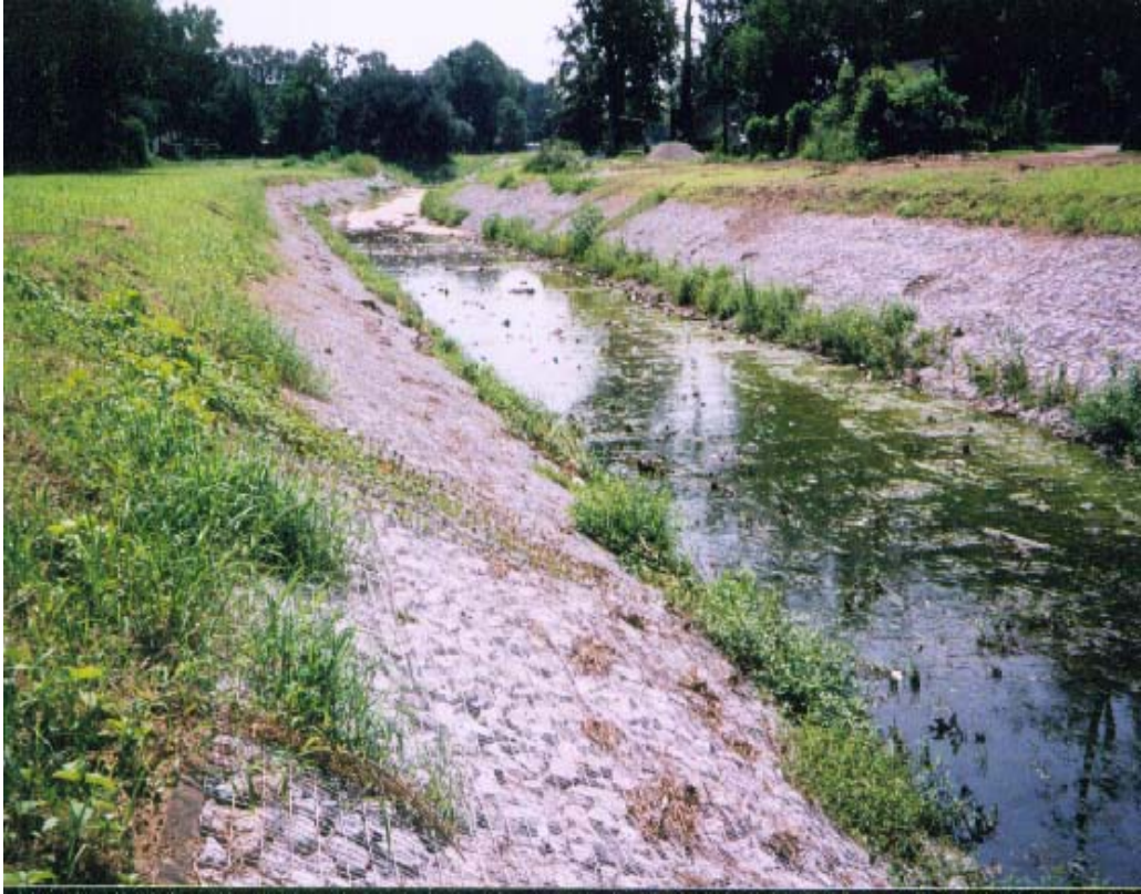
Figure 2.1: Gabion Mattress Channel Lining
