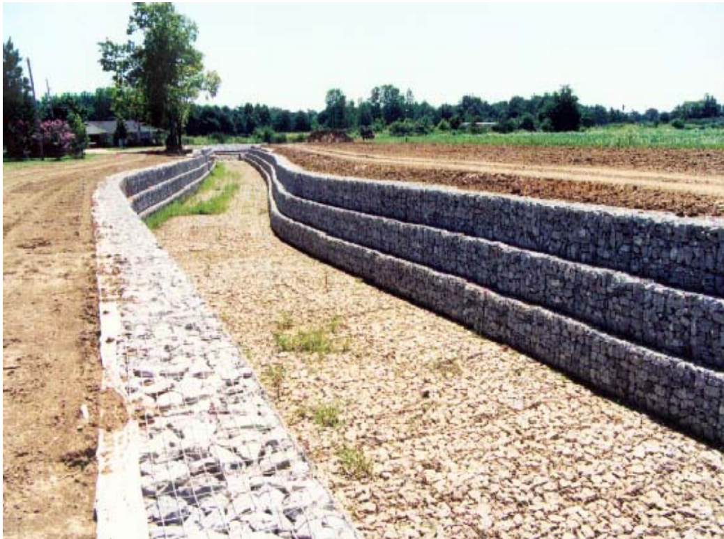
Figure 2.2: Gabion Walls for Flood Control and Bank Protection
